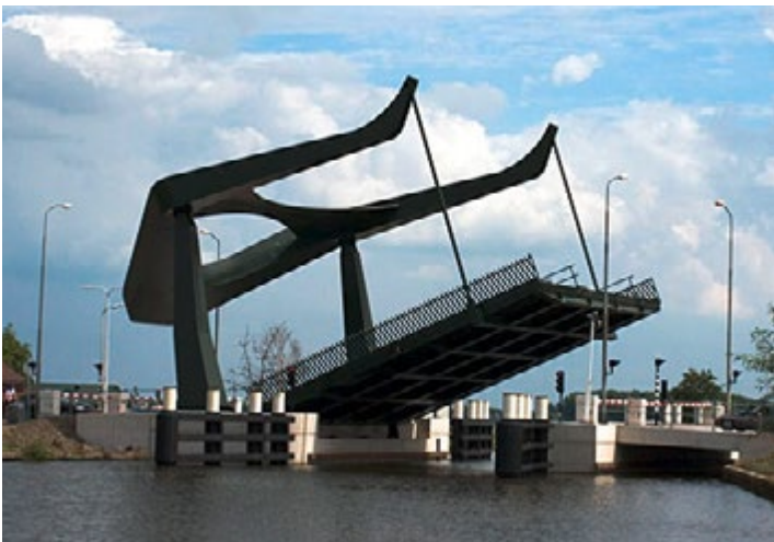
OPENING BRIDGE „PRAYER OF SHADOW“: The spectacular bridge over the Amstel is coated in RAL 6007 Bottle green. Within the space of a minute, this high-tech-bridge in Vrouwenakker (south of Amsterdam) can be raised or lowered.
